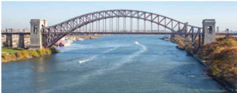
Above: Hell Gate Bridge, November 2022 Photo Credit: Trent Reeves/MTA
