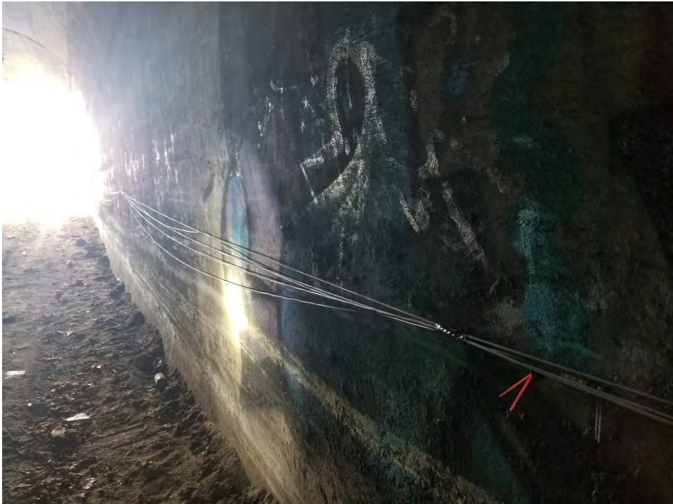
Picture 6 – Inactive tunnel, looking south
