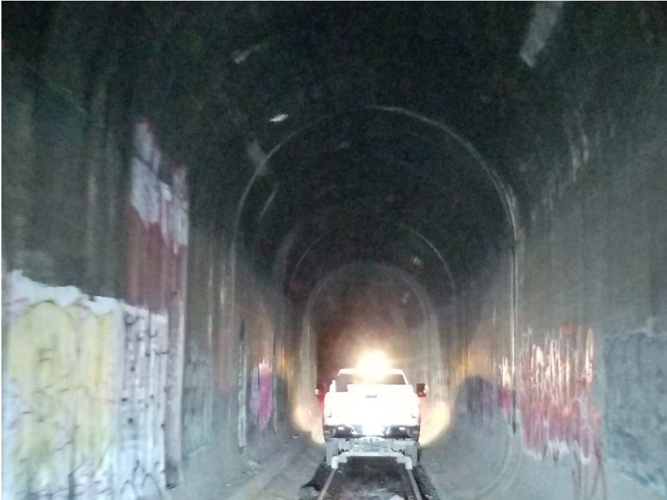
Picture 2 – View from inside active freight tunnel, looking south
