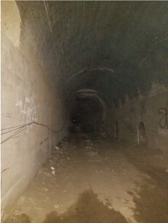
Picture 9 – Inside out-of-service tunnel on west side
