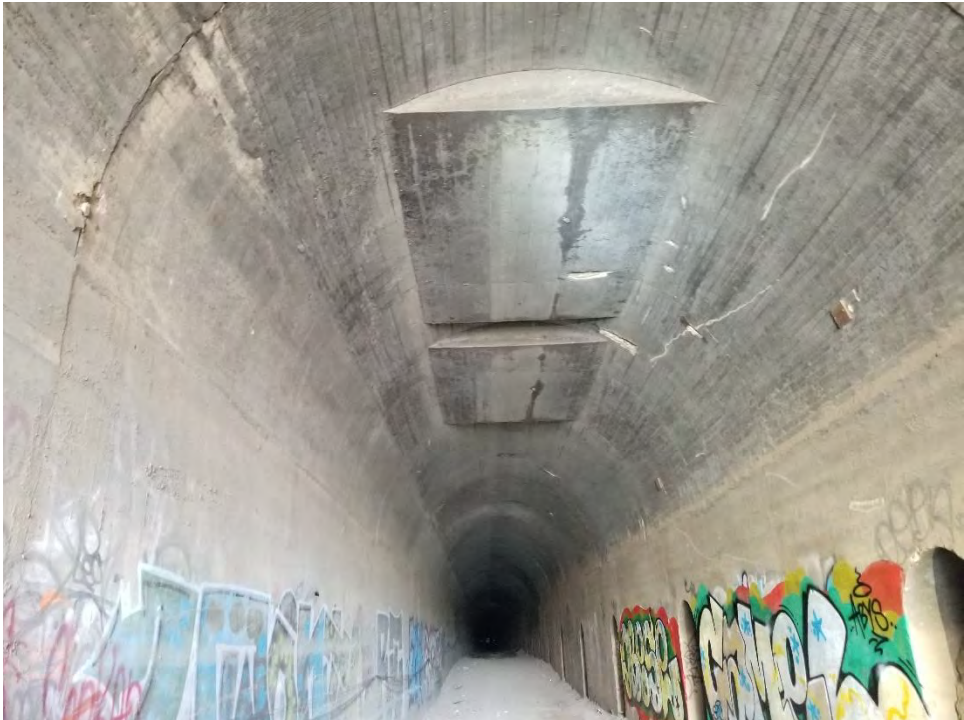
Picture 4 – Out-of-service tunnel, looking north
