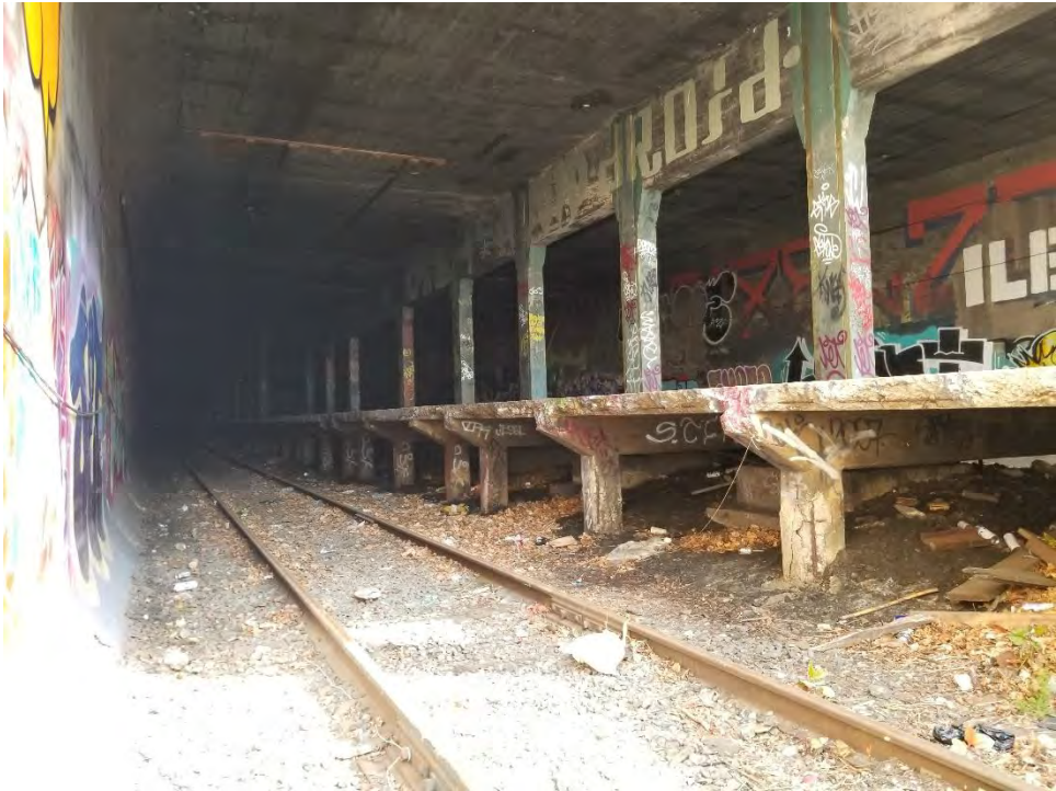
Picture 12 – Abandoned transit platform at south end of tunnel
