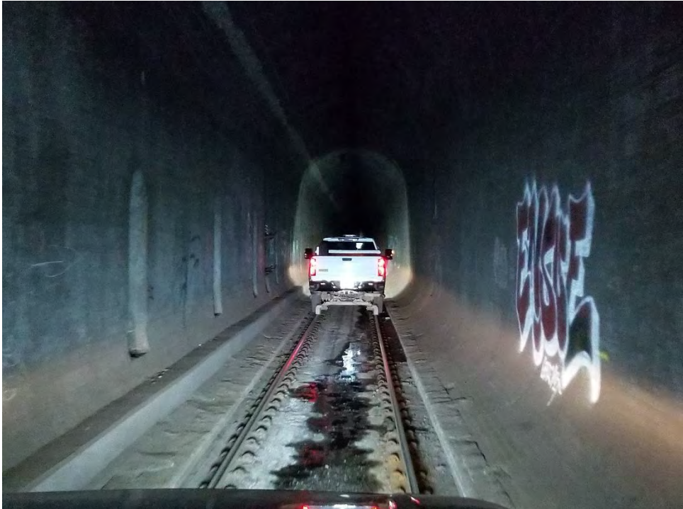
Picture 3 – View from inside active freight tunnel, looking south
