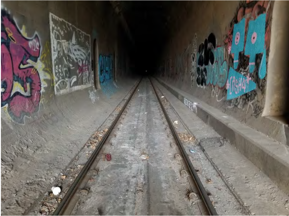
Picture 11 – Inside existing freight tunnel direct track fixation
