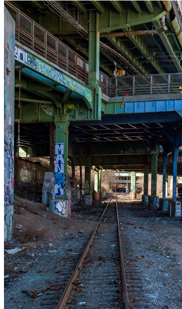
IBX Route conditions under 5th Avenue & Interstate 278/Gowanus Expressway
